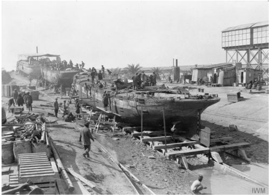
Above: Magil Docks Slipway on the Euphrates
